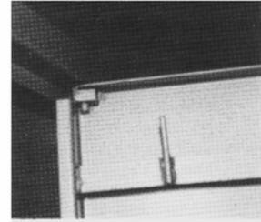
Cabinets with exposed hinge barrels and those with piano hinges which have been fitted using rivets require anti-prise plates.
