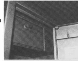
The lock mountings to be welded to the door of the cabinet, ensuring the lock is so secured to prevent its movement if attacked. Two locks are required on full length rifle cabinets fitted at  $\frac{1}{2}$  and  $\frac{2}{3}$  of the doors length
