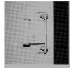
Fastenings must be appropriate to the size and structure. 'Rawl' and expanding bolts should be utilised in stone, brick and concrete. Coach screws and bolts for timber joists. The cabinet manufacturers will usually include recommendations for fixing devices
